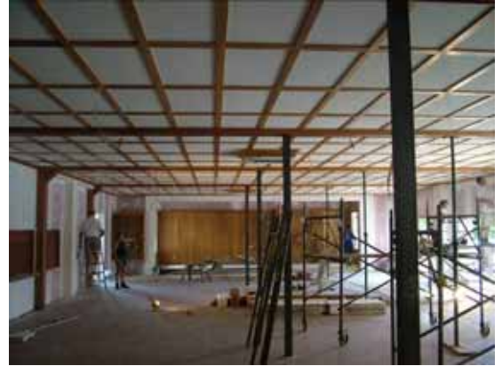
Completing the attractive new ceiling in the newly extended Dining Room
