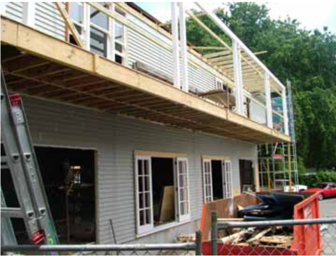
Excellent progress with the Dining Room extensions.
