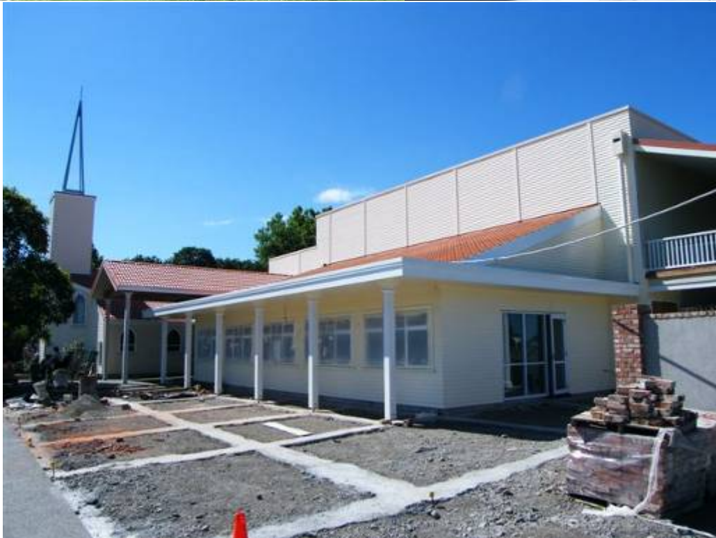
The Performing Arts Centre nearing completion
